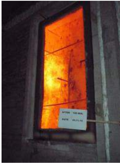
2 Fully Glazed 120 Minute Fire Rated Door at the end of Fire Test
