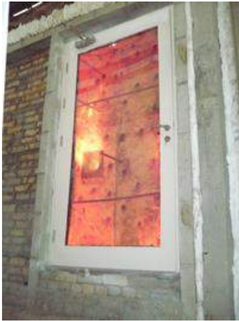
1 Fully Glazed 120 Minute Fire Rated Door at the start of Fire Test
