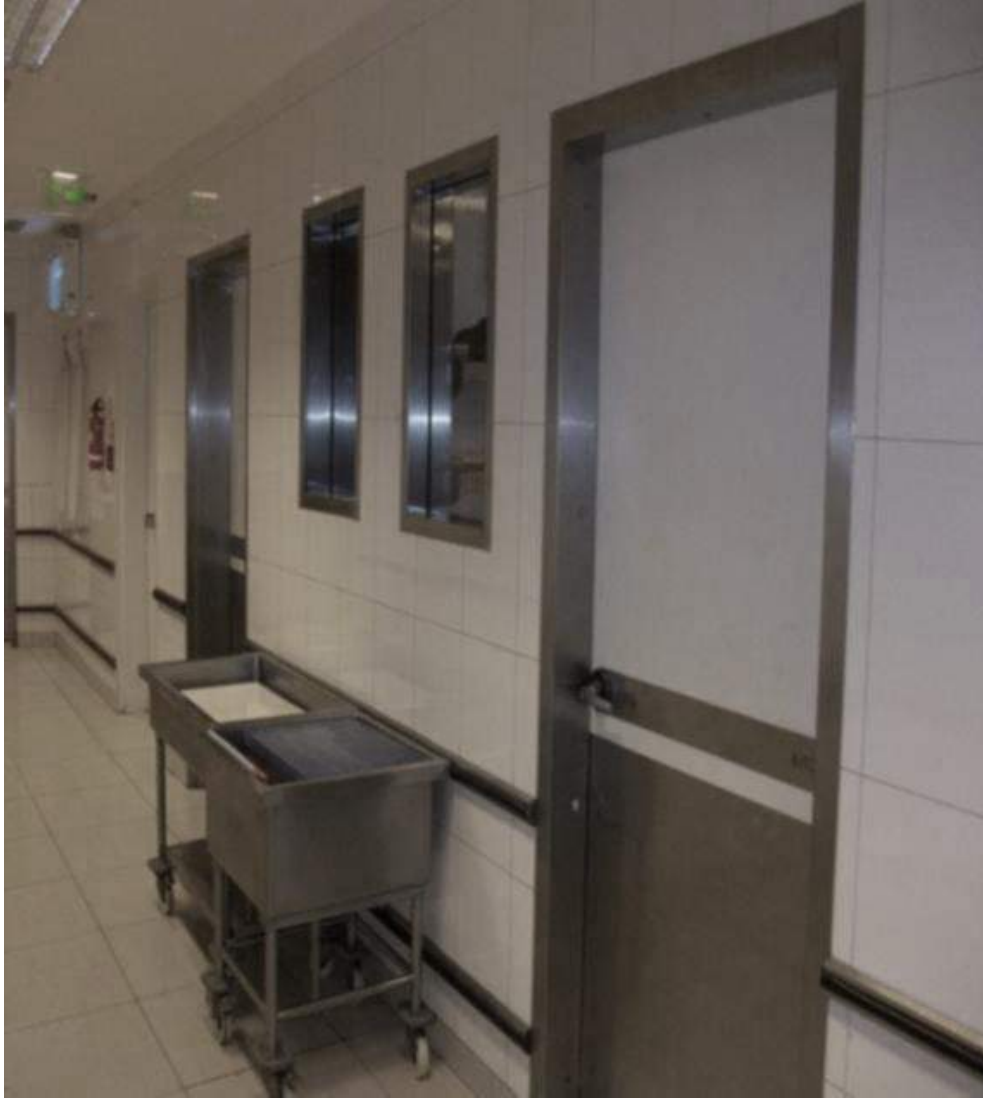
1 Stainless Steel Kitchen Doors & Windows at the Trident BKC
