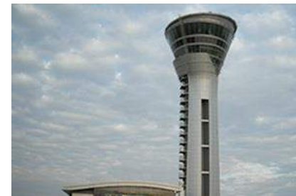
3 ATC Tower Delhi International Airport
