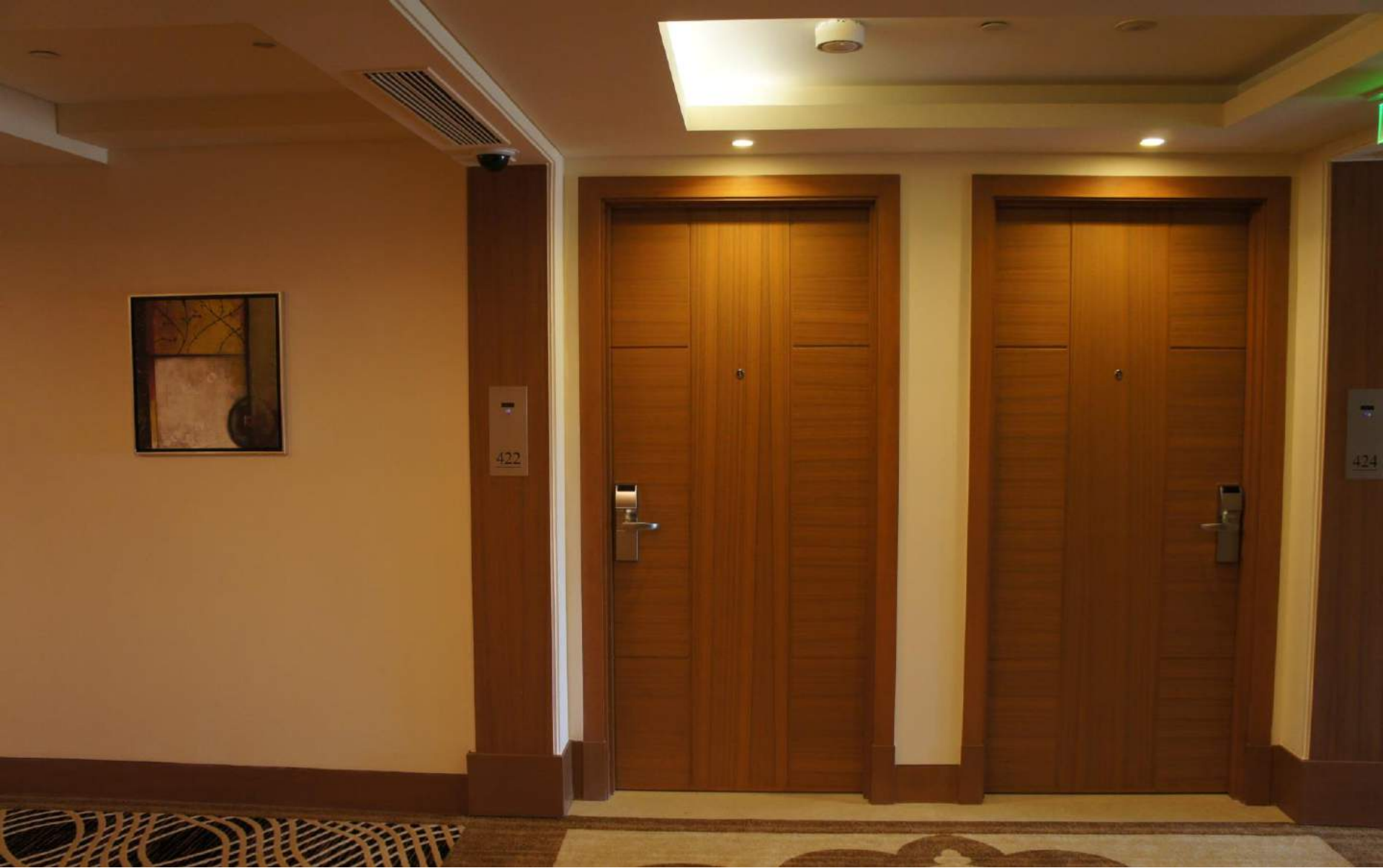
1 Veneered and Polished 120 Minute Fire Rated Timber Doors for Guest Room Entrances
