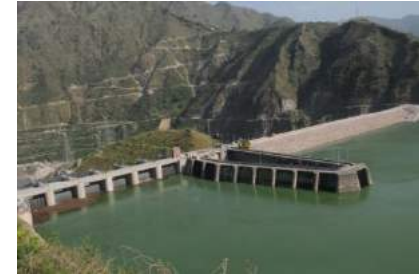
3 Koldam Hydro, Himachal
