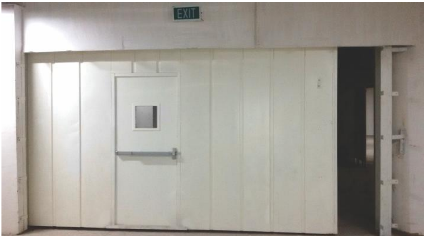
120 Minute Fire Rated Sliding Door with Emergency Exit Wicket Door with Vision Panel and Panic Device
